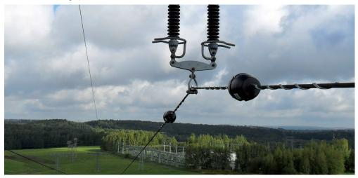
Sensor nodes of the ASTROSE<sup>®</sup> system monitore power lines in Germany. They collect data about inclination and oscillation of the lines, temperature and current. Photo © Fraunhofer ENAS | Download: www.enas.fraunhofer.de/en/news\_events/presse\_uebersicht.html
